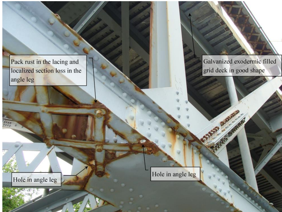
Figure 32. Photo. Annotated picture of riveted lower truss chord connection.
