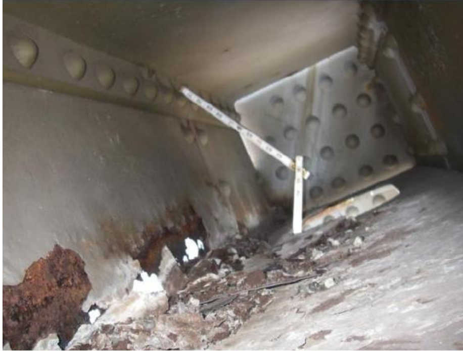
Figure 33. Photo. Inside of built-up box member.
