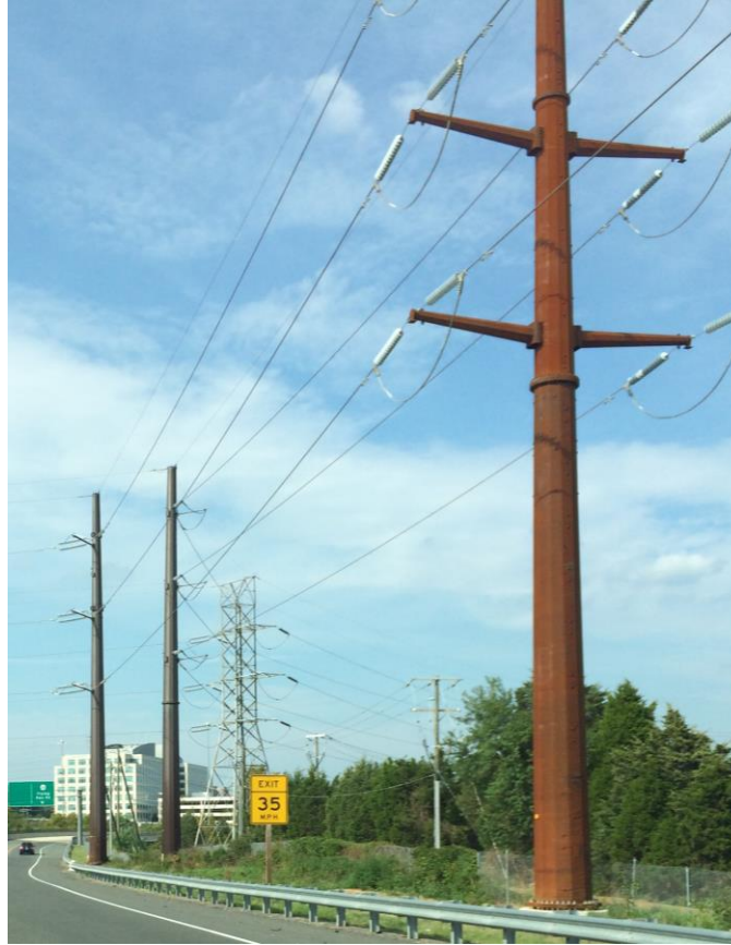
Figure 8. Photo. Different color of rust patina in new transmission tower (close) and older (far).
